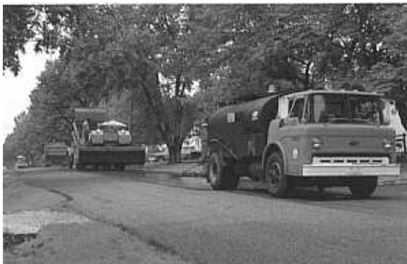
Lightweight aggregate bonds uniformly to asphalt to create a safe and durable road surface.
